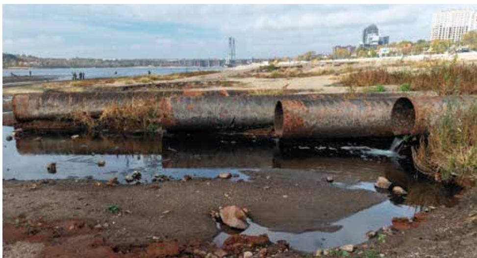
Photo 3.4: Discharge of wastewater from local sewage system to Dnipro River in Zaporizhzhia - near the site L1 Central beach. (Photo: Majda Slámová)
