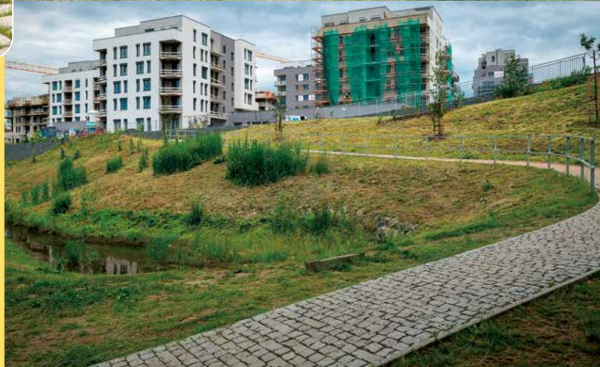
**A residential area was developed on a brownfield site, transforming it into 23 apartment buildings with green spaces that effectively manage rainwater. The project features a cascading system of trenches and polders for water retention and irrigation of greenery, reducing runoff and flood risks while enhancing the local microclimate.**
