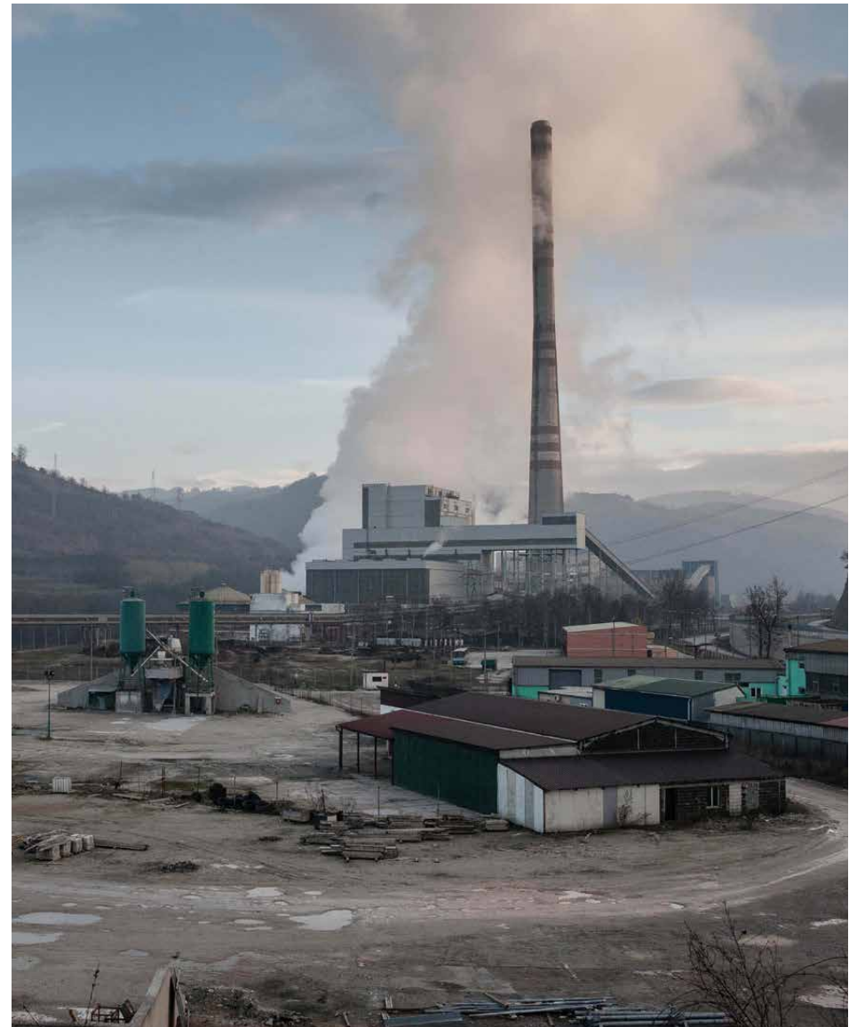
Photo 4.7: In 2014, the Kakanj brown coal power plant was among the largest sources of pollution in the Zenica area. Photo: Martin Plocek, Arnika, 2014
