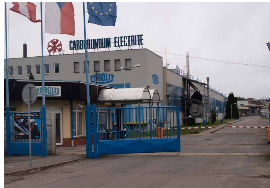
Photo 4.23: Carborundum Electrite in Benátky nad Jizerou in January 2015. The small vent at the hall's beginning is the preliminary unit's chimney for the discs' production using naphthalene. It is no longer there today, just like the planned production with naphthalene. Photo: Jindřich Petrlík, Arnika, 2015
