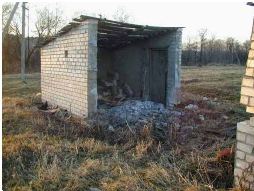
Figure 14: Small storage area of the mixture Polho made of WI fly ash. Site near village Belaruchi, Belarus in 2007. Photo by Center of Environmental Solutions (CES), Belarus.
