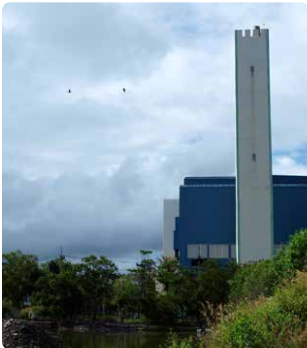
Figure 16: MSW incinerator in Phuket, Thailand with small pile of ash in front. Photo by Jindrich Petrlik, Arnika, December 2010.
