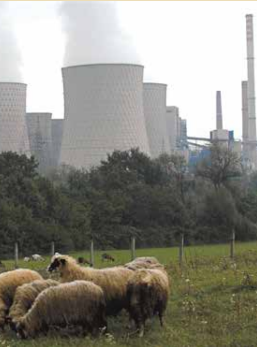
Tuzla thermal power plant Photo © Ondřej Vlček
