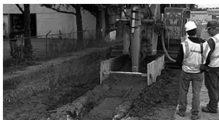
Figure 10: Combined trenching and slurry insertion
