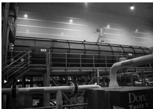
Figure 15: The Indirect Thermal Desorption Unit (ITDU) at Spolana Neratovice, Czech Republic.
