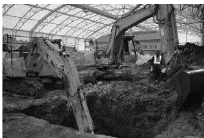
Figure 8: Interior of Odour Control Enclosure during excavation. Source: Australian Federal Government (2013)
