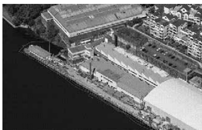
Figure 7: Remediation with Odour Control Enclosure and treatment train. Source: Australian Federal Government (2013)
