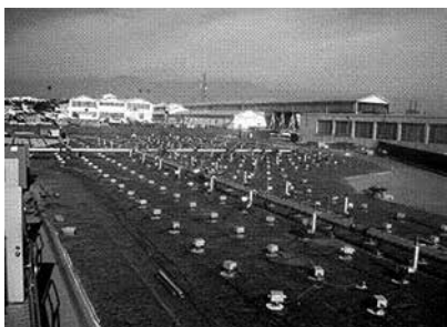
Figure 12: Full-scale ISTD operation on organic compounds contamination in the USA. Source: Merly and Hube (2014)
