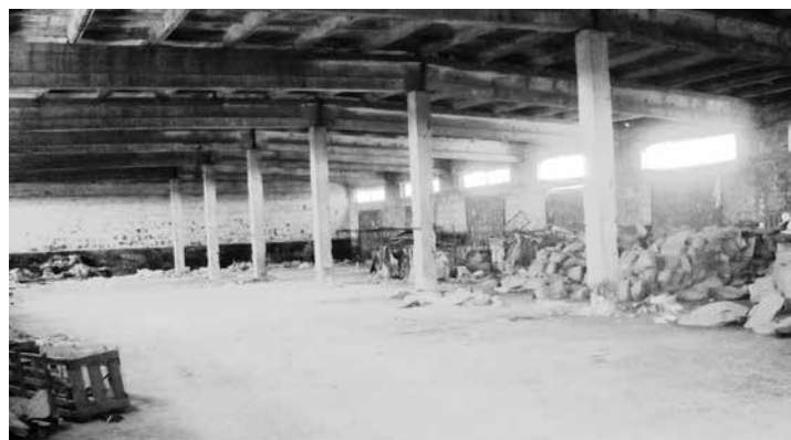
Figure 5: Interior of the building of the big storage in Jرات. Author: Z. Honzajková
